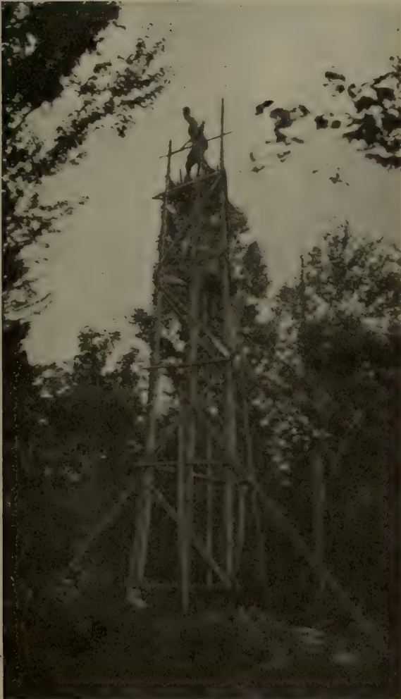
FIG. 19. Forty-foot Tower built on trees in place.
